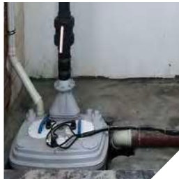
-1. kat zeminine kurulan SANICUBIC 2 VX
